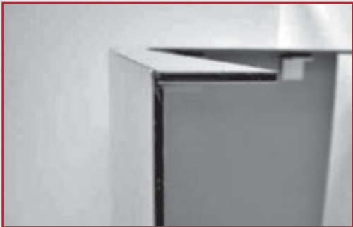
Cope at Edge of Panel
