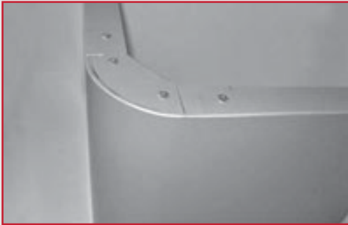
Corner Panel with Gusset & Filler Plate
